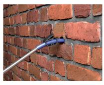
Once ready to fill, slip a clamp over the exposed hose, then push fit the steel pipe into the open end. Switch on the compressor and proceed with pumping.
