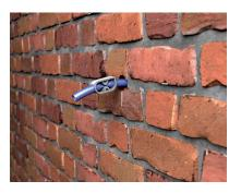
11. After a few minutes, fasten the clamp before turning off the compressor. It is advisable to remove the hose from the threaded tube 2-3 hours after installation. Wash any excess grout off with clean water, then fill the holes with SureFill flexible pointing mortar and colour match the masonry with SureStain.
